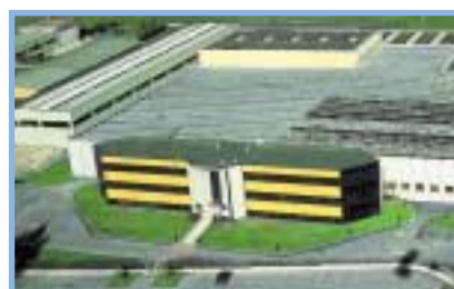
Tool- and manufacturing plant in Caprino (It)
